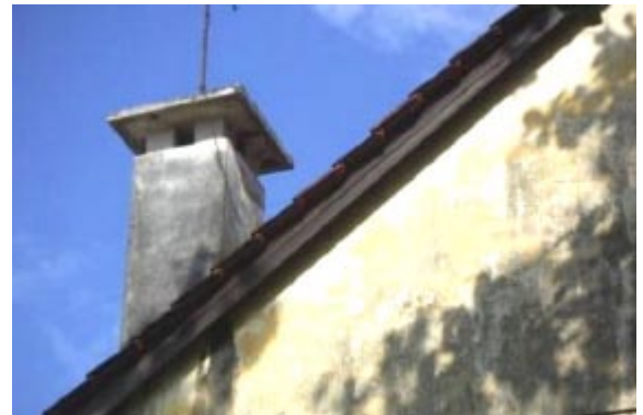
Chimney for the cooking stove below
