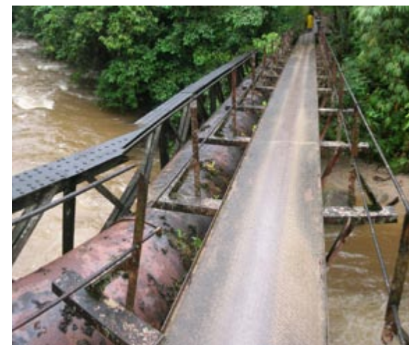
Metal bridge beside the pipeline.
