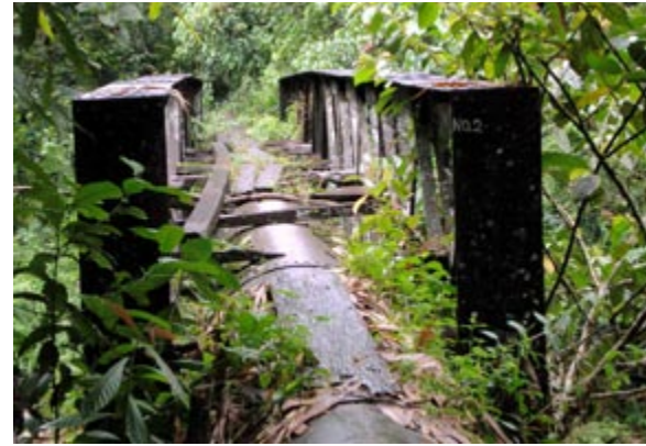
Pipeline as the bridge.
