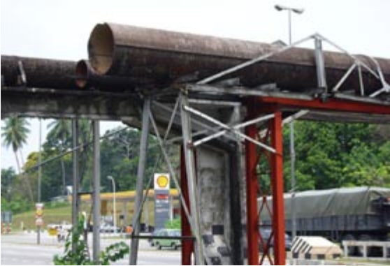
Cut away pipe over the main trunk road in Gopeng.
