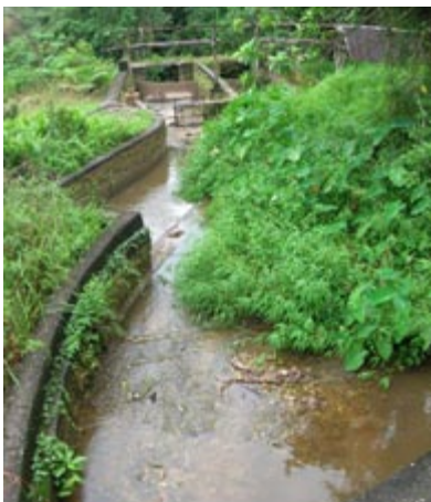
Water intake at the dam.
