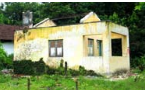
Roof tiles salvaged (see details of roof tiles, pg 3).
