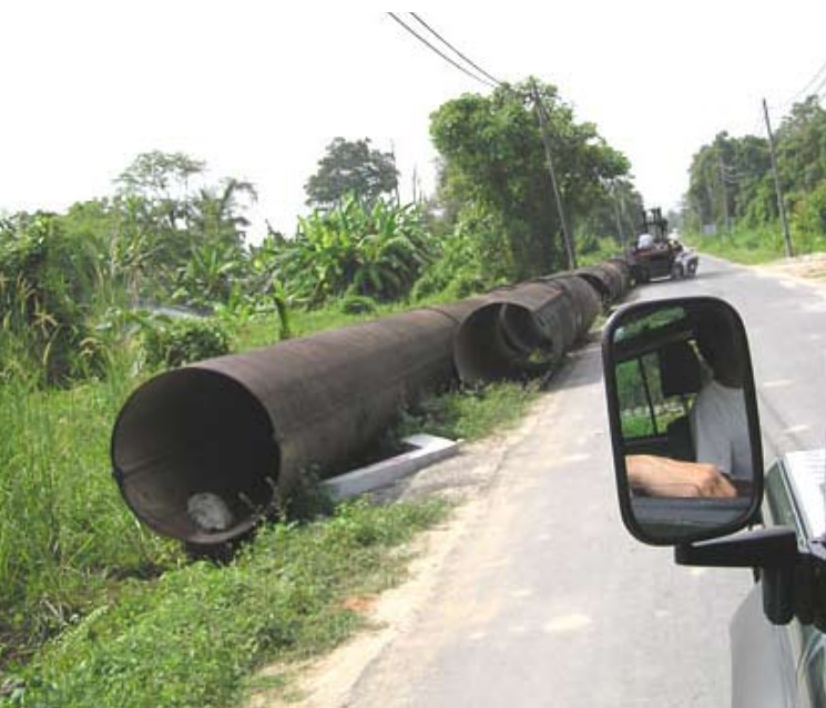
The dismantling of the Kampar Pipeline in Gopeng. Photos : Charlie Chong
