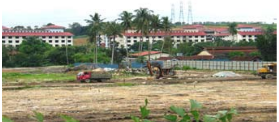
Demolished and levelled - hospital buildings in the background.
