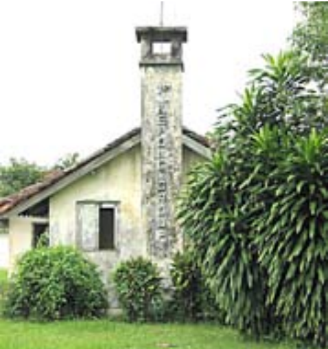
Building donated by Kepong Group? note the inscription on the chimney
